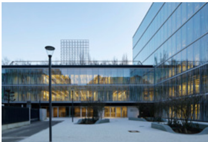
The BIMSB building at the MDC site in Berlin-Mitte © Noshe
